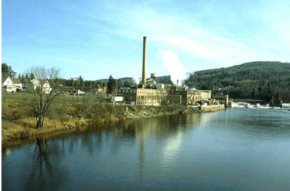
Dam and Generating Station in Gilman, VT on the Connecticut River (© B.B. Greenbie)
